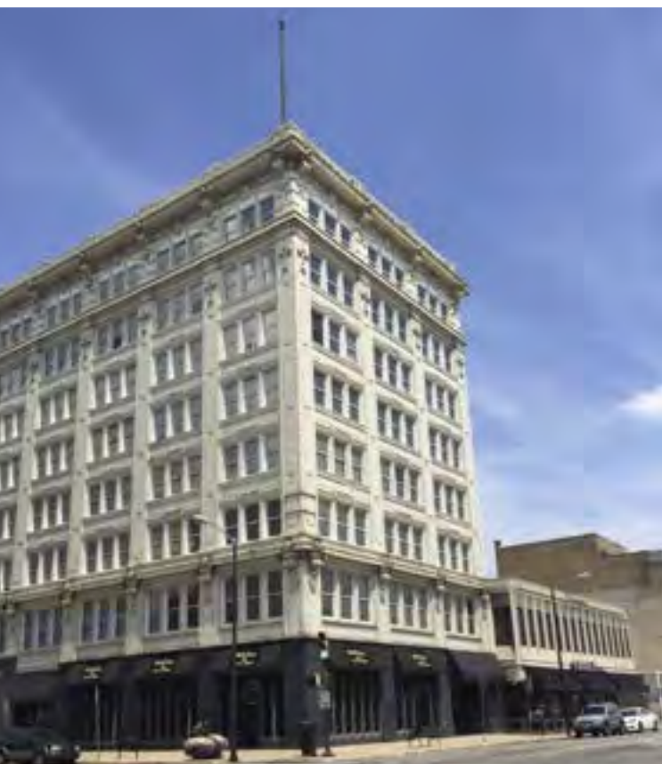
p41 SLATED FOR RENOVATION The historic JMS Building in downtown South Bend is named after John Mohler Stuebaker, one of the brothers behind Stuebaker Corp.
