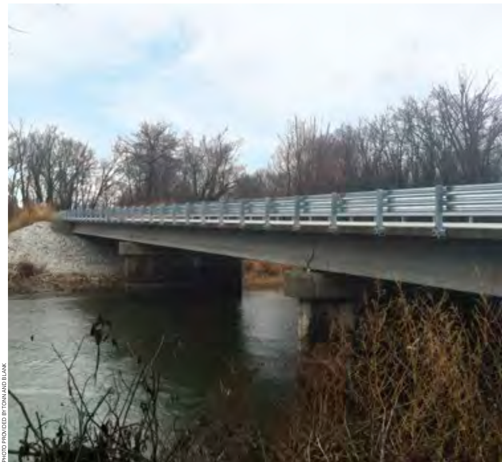
BUILDING BRIDGES Tonn and Blank Construction of Michigan City completed this span taking County Road 500 East over the Kankakee River in Porter County.
