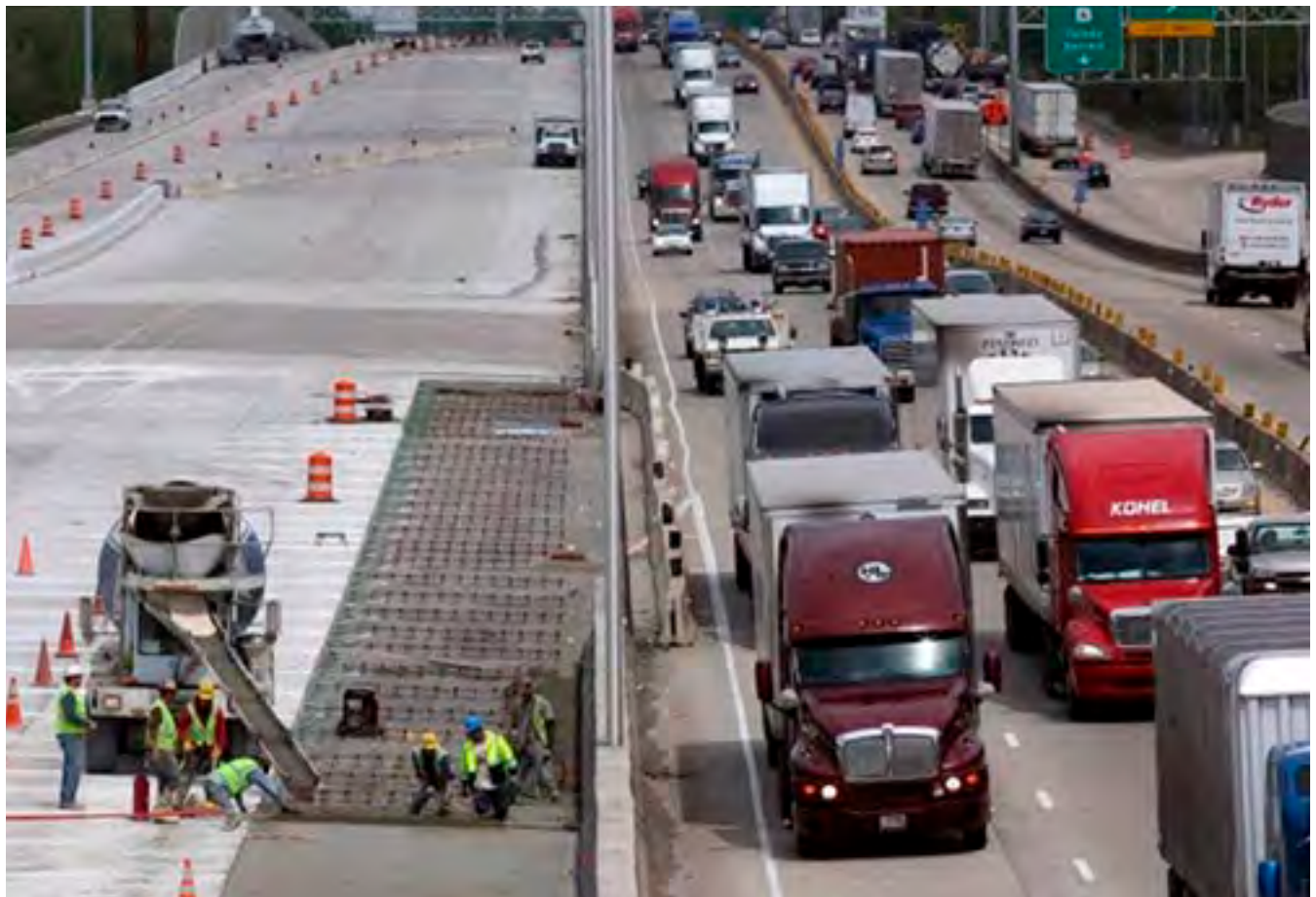
REHABBING THE BORMAN EXPRESSWAY A $700 million project has made the road more safe and more efficient.
