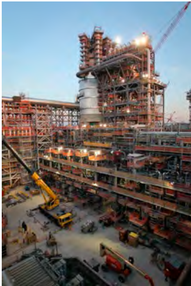
MODERNIZATION The BP Whiting refinery is reconfiguring its largest crude distillation unit to process heavier crude.
