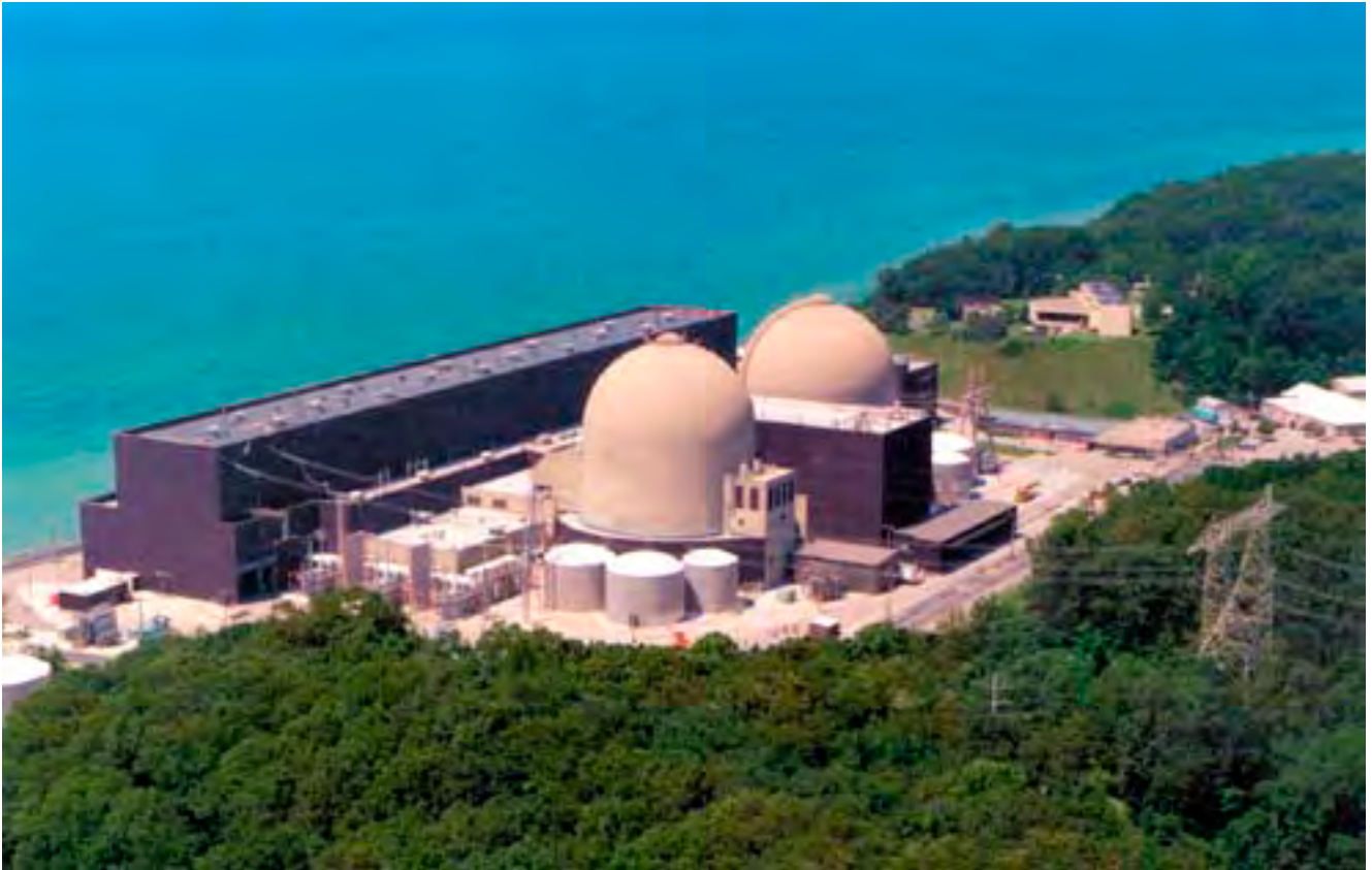
JUST ACROSS THE BORDER The Cook Nuclear plant in Bridgman, Mich., is operated by AEP Corp.
